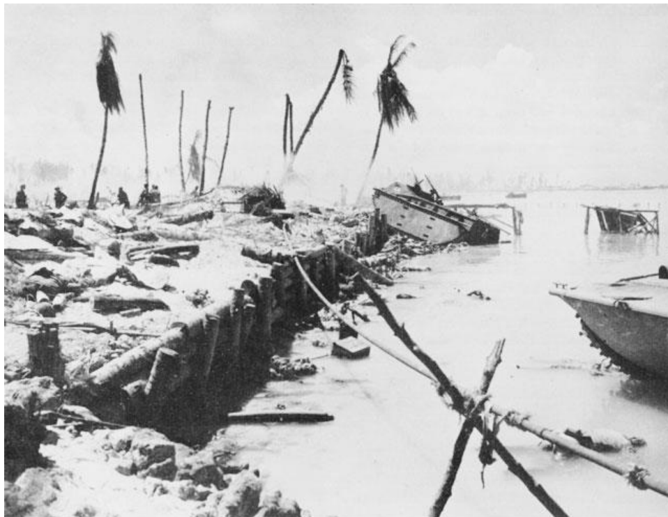
View along the North Beach showing the seawall and a pillbox.
